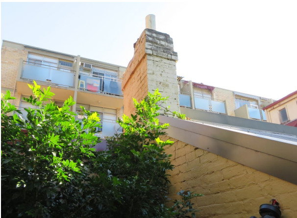
Figure 16 – View north to the later south façade of 96 Brougham Street. the original party wall is evident below the eaves line of 98 Brougham Street. Original joinery to the front of 98 Brougham.
