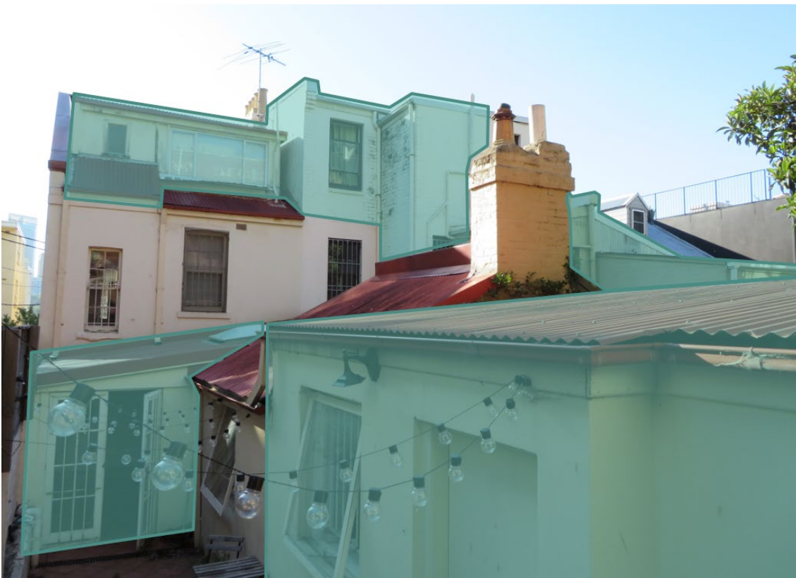
Figure 9 - Rear elevations of 96 – 98 Brougham Street showing later fabric shaded blue.
