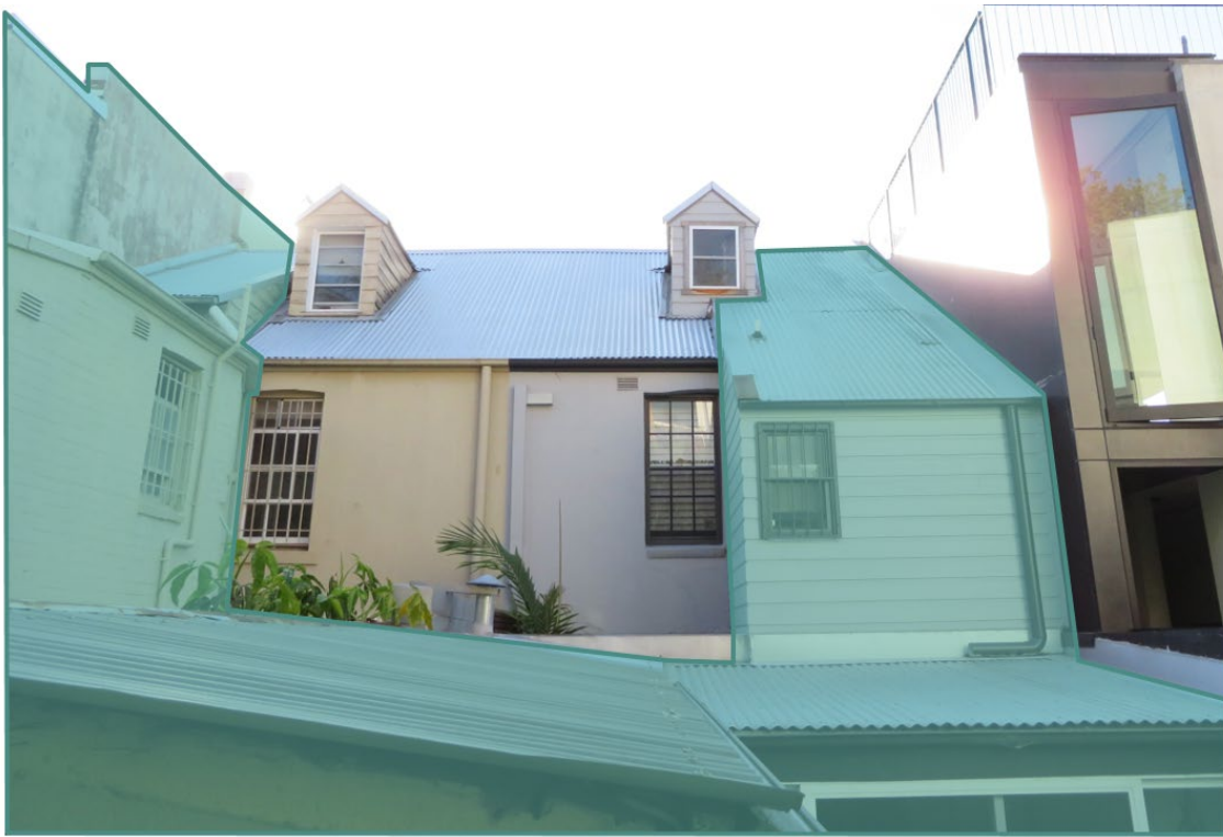
Figure 8 - Rear elevations of 92 – 94 Brougham Street showing later fabric shaded blue.
